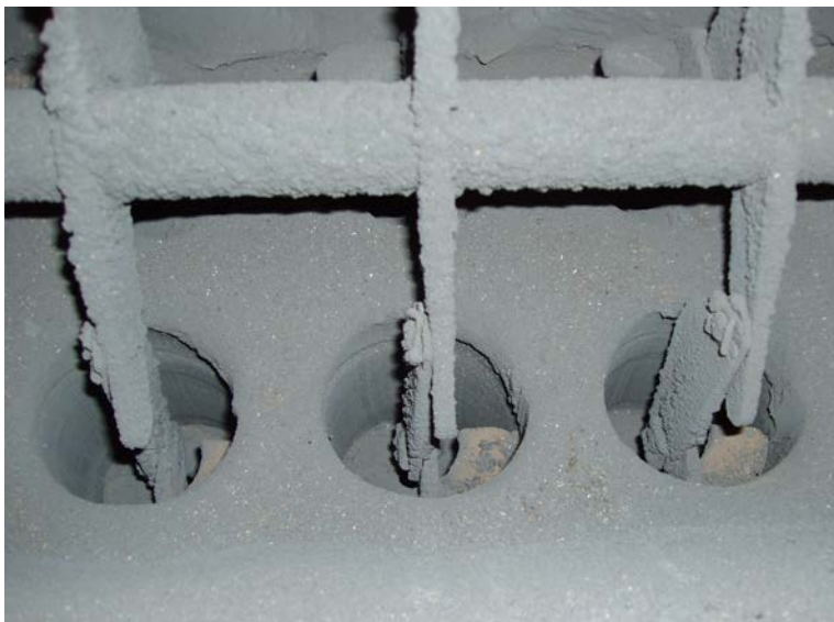
Figure 21: Automatic cleansing of the heat exchangers based on spirals (left) or compressed air (right).
