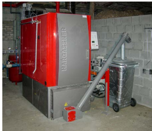
Figures 23 and 24: Ash container and discharge of ashes through a feed screw.
