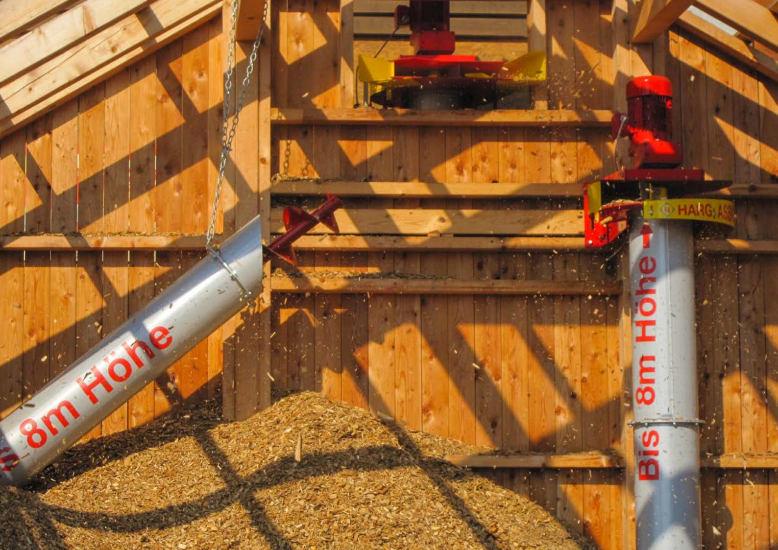
Figure 12: Filling system with screws for supply of wood chips to the silo.
