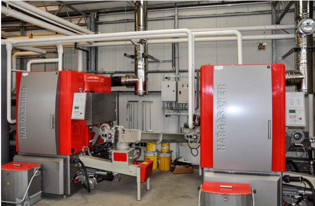
Figure 16: Configuration of biomass boilers in cascade configuration.
